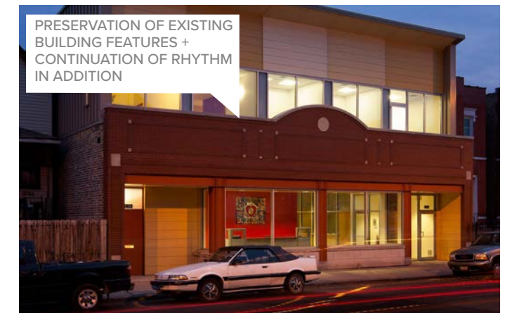
Adaptive Reuse - Addition to Single Story Building Spanish Coalition for Housing Offices Source: LBBA
