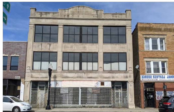
Industrial / Manufacturing Buildings 4613 N Clark St - Vacant Property
