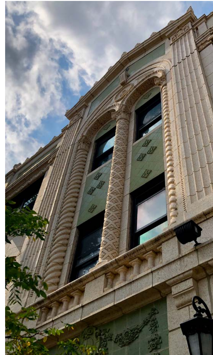
Historic Façade and Massing
