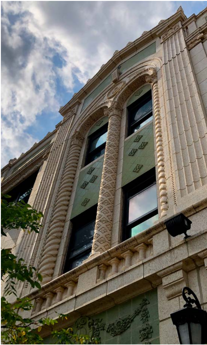
Historic Façade and Massing
