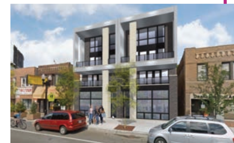
4645 N CLARK ST (2021 - UNDER CONSTRUCTION)
