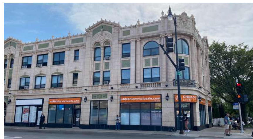
Issel Building (c. 1929) 4532-4558 N Clark St – Landmark
