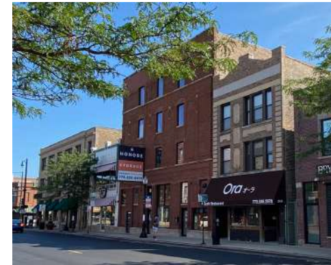
H Honore Storage – 5147 N Clark Use: Residential storage warehouse
