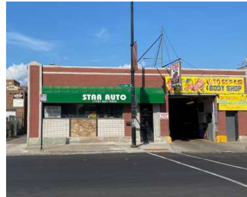
F Star Auto Repair and Body Shop – 5000 N Clark Curb cuts on Clark Street Insufficient storefront transparency
