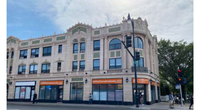
Issel Building (c. 1929) 4532-4558 N Clark St – Landmark
